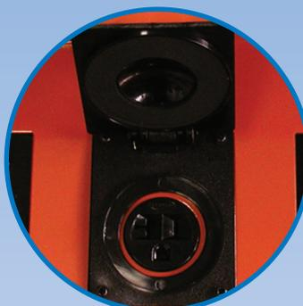
All outlets are protected with weatherproof covers and are circuit breaker protected against overloads. The 20 Amp outlets have additional GFCI protection for added safety.
