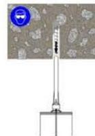
11. Select the steel anchor element ensuring it is free from oil or other contaminants, and mark with the required embedment depth. Insert the steel element into the hole using a back and forth twisting motion to ensure complete cover, until it reaches the bottom of the hole. Excess resin will be expelled from the hole evenly around the steel element and there shall be no gaps between the anchor element and the wall of the drilled hole.
