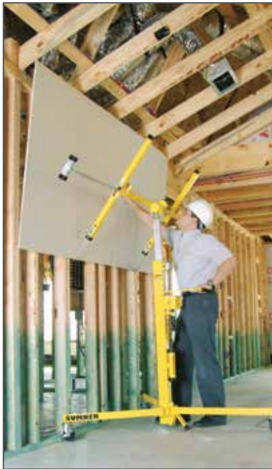
Steering leveler provides optimum positioning.
