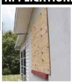
Direct mount permanent anchors for quick and easy installations for metal and plywood panels to wood, hollow block and concrete.
